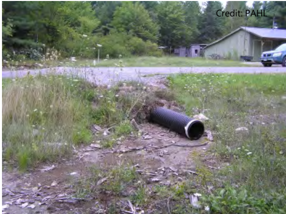
Culvert under Hyde Lake road installed during a 2010 infrastructure project by the Theresa highway department.
